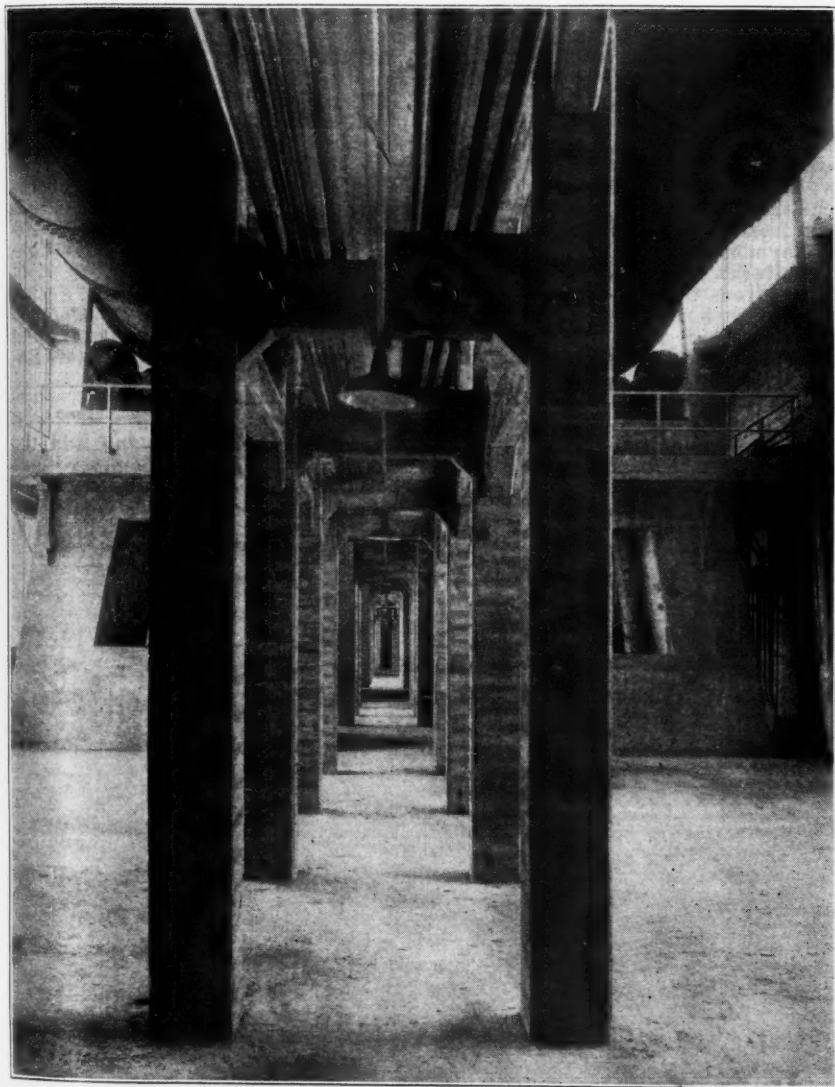
Interior View in Kiln Room Showing Type of Structure
